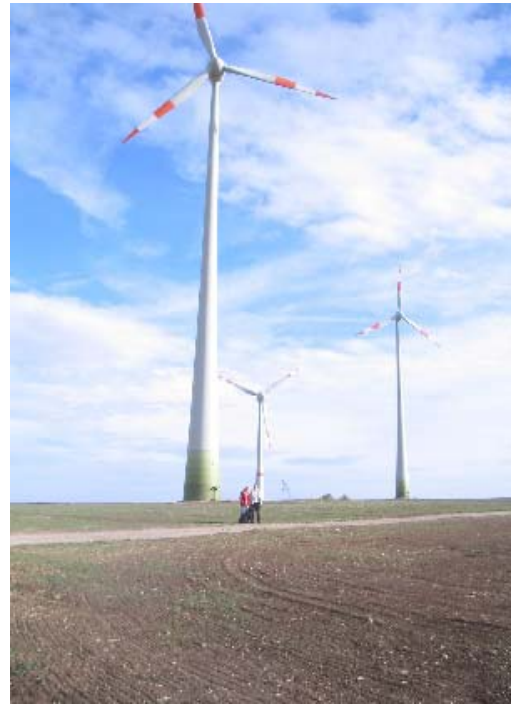
Windpark: Druiberg, near Dardesheim
