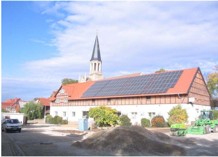
Dardesheim utility building
